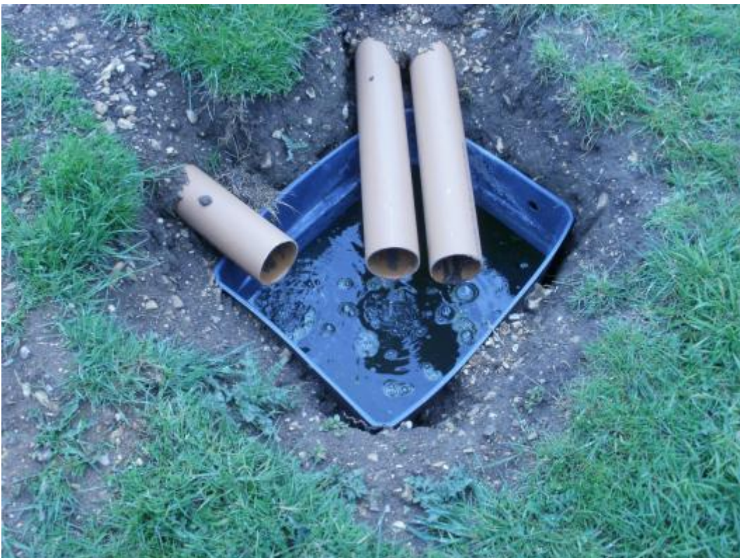
Figure 4-25 Tailwater monitoring chamber
