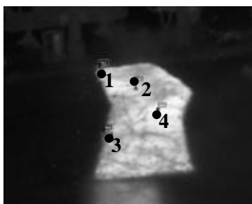
Figure 9: Thermal image of patch repair immediately after compaction on repair site 2
