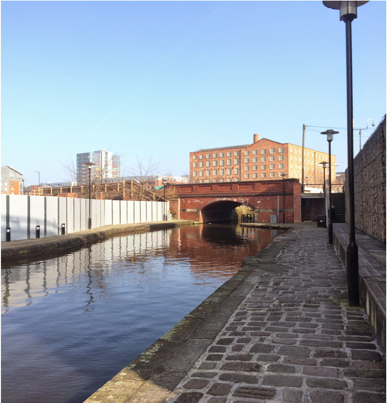
Figure 3: The Bridge © the author, 2014.
