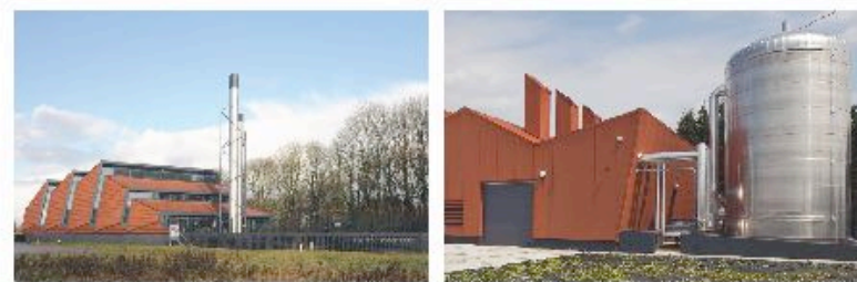
Eco Zathe Heat and Power Plant, Leeuwarden
