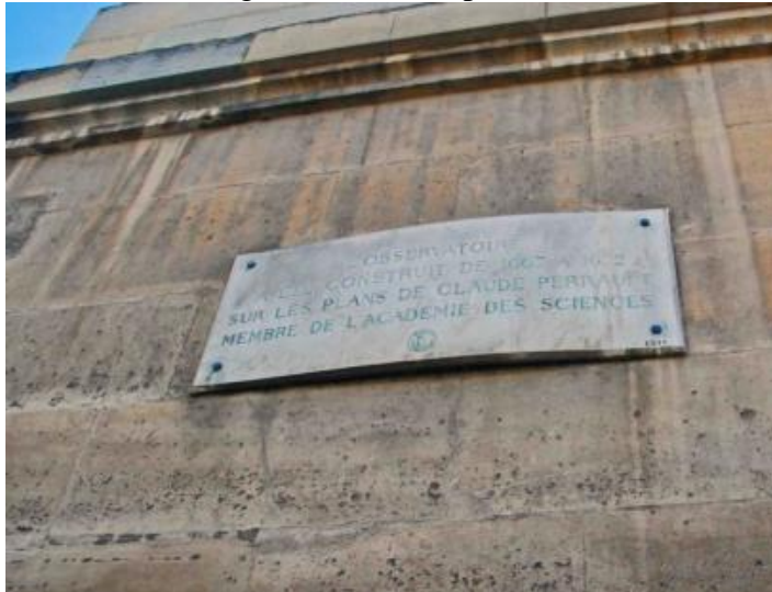
Fig. 1. A commemorative plate on the Observatoire de Paris (14e arrondissement), fixed in 1672 at the time of the inaugural ceremony, but now distorting due to surface weathering processes. “Observatoire construit de 1667-1672 sur les plans de Claude Perrault 1 , membre de l’Académie des sciences” The wall is comprised of Lutetian limestone (Eocene) and is full of the molds of molluscan shells. © P. De Wever
