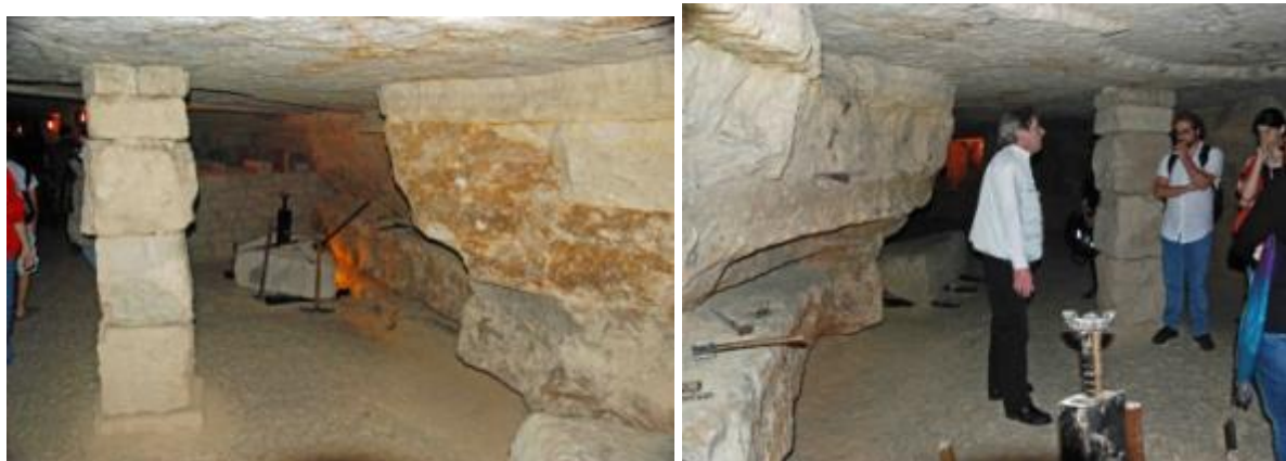
Fig. 04- Underground quarries below Cochin hospital, Paris. The pillars, bed rock and tools bear witnesses to the work used to extract these stones for building Paris. © P. De Wever
