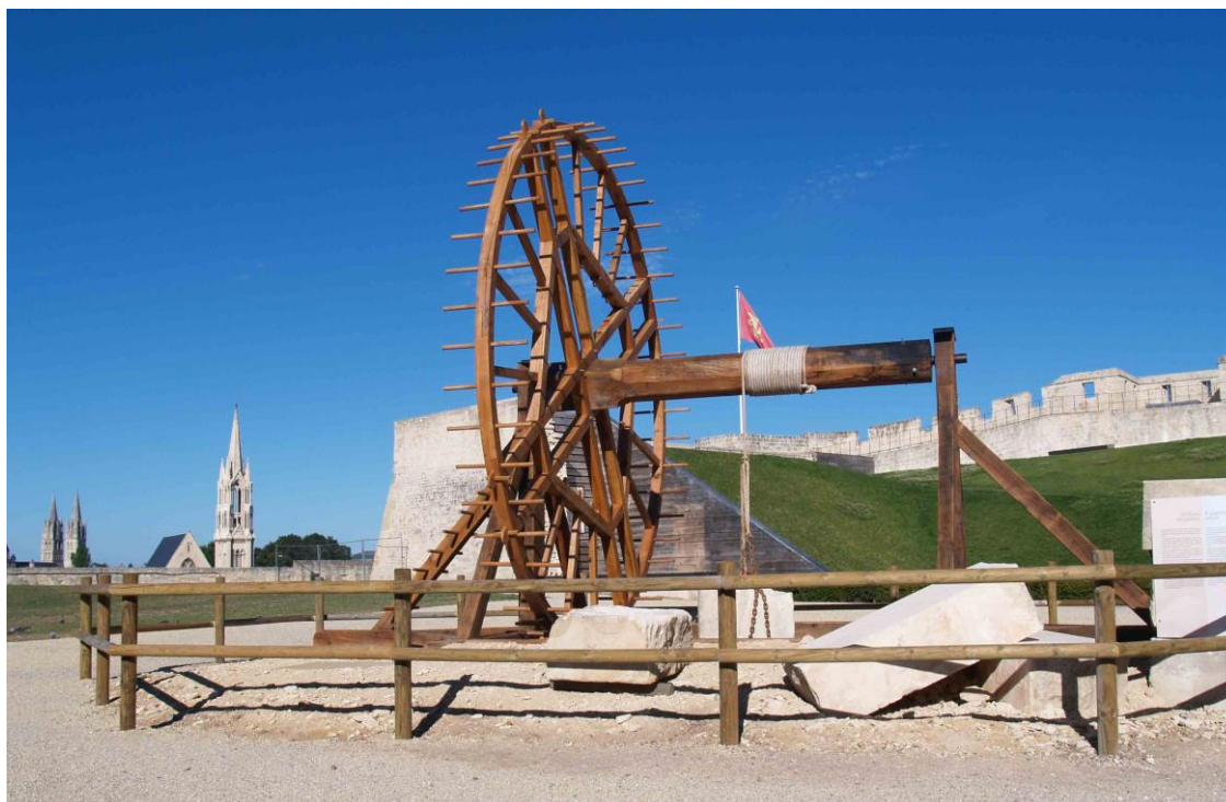
Fig. 14- Winch used to bring to the surface heavy blocks of Pierre de Caen from underground quarries - note the white colour of the stone © D. Peeters
