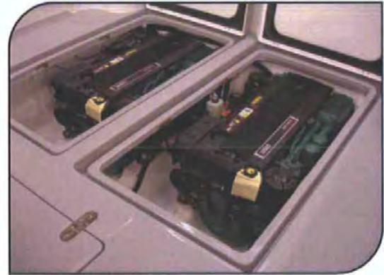
High parity with real-life geometry: essential due to complex inter-relationships between components and equipment.
