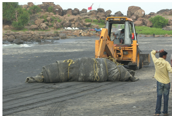
Figure (2.1). Kovalam ASR, Kerala, India. September, 2010. Photograph showing the clear up of the beach after the first monsoon post-construction of the Kovalam ASR; one of the geotextile sand bags is washed ashore.
