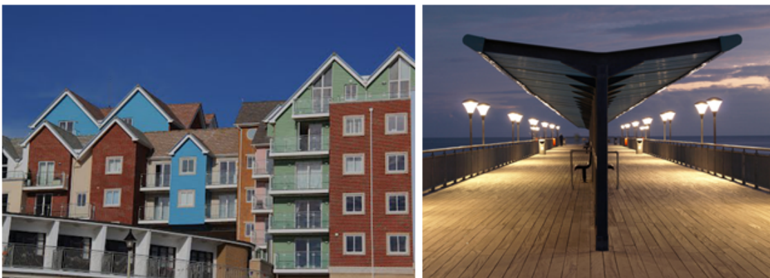
Figure (4.4). (a) The new build Barrett's Homes apartment complex (Honeycombe Beach flats) built on the old car park, and (b) The shortened and renovated Boscombe pier, lit up in the evening.
