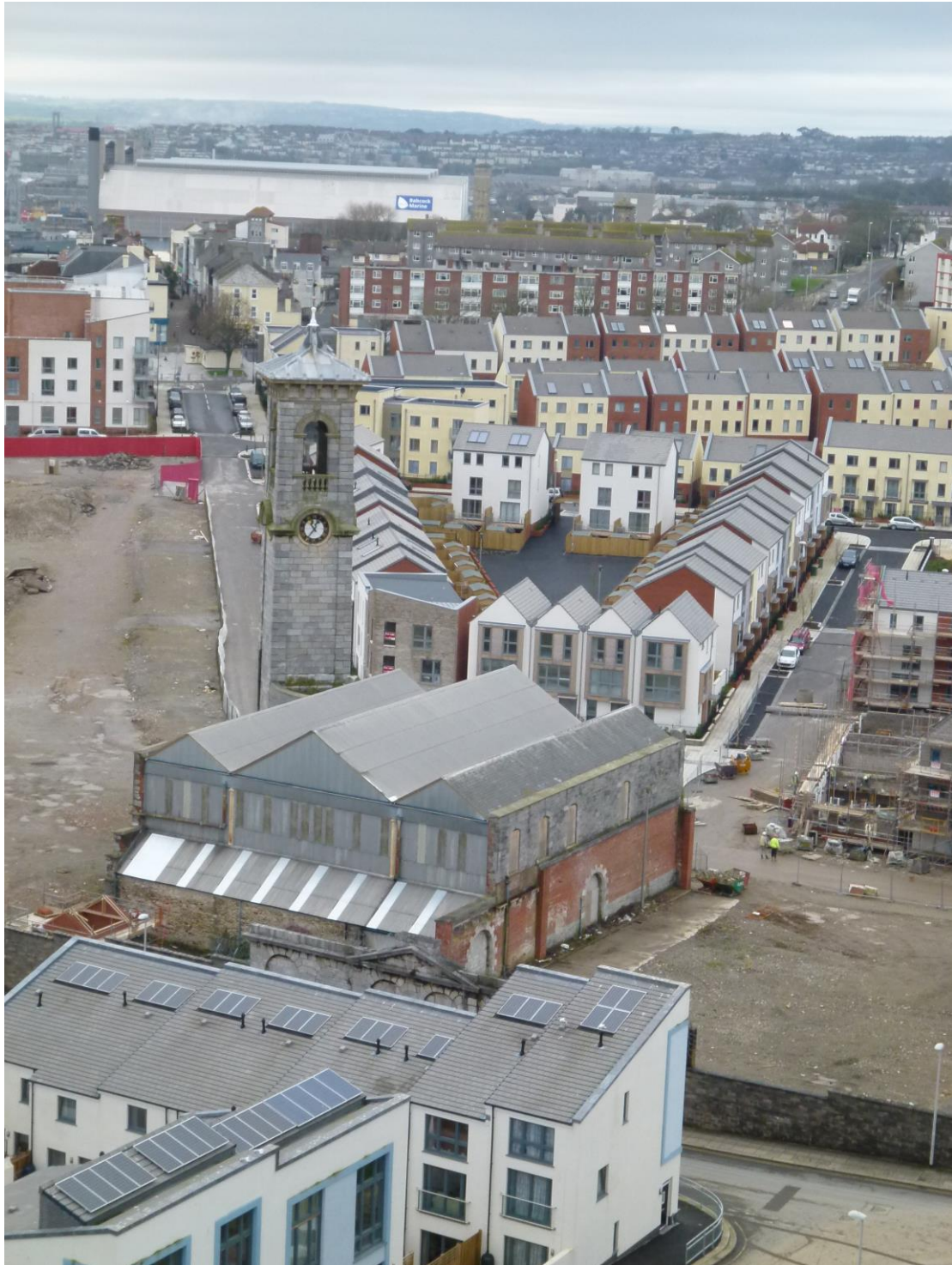
Figure 8. Redevelopment of the South Yard Storage Enclave in March 2012. Before the Second World War, this area was the site of the town centre of Devonport. It was requisitioned by the Navy in 1952. The enclosing dockyard wall is just visible in the bottom right hand corner of the photograph. New mixed use development by Redrow is taking shape on the former storage enclave. The old market building (adjacent to the clock tower) is being retained within the layout of the new development and has now been purchased by Plymouth City Council as the basis of a community-led regeneration scheme.
