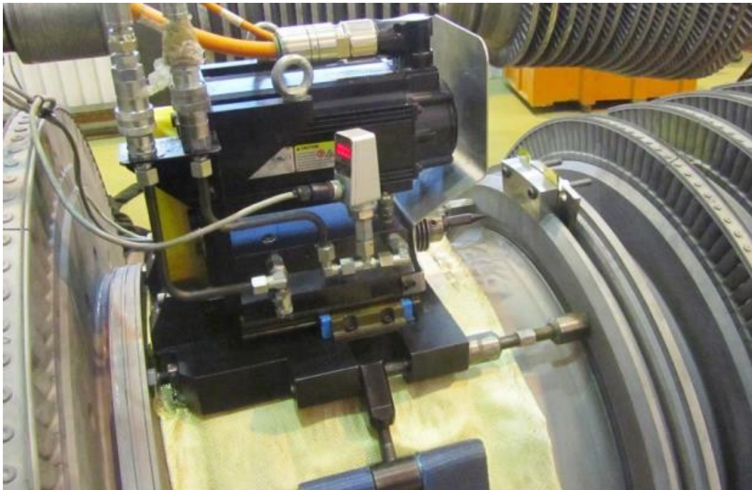
Figure 20 Illustration of the bespoke FHHP platform in position on a stream turbine rotor. It uses the registered WeldCore® process and in this case, is being used to extract samples for creep damage analysis.
