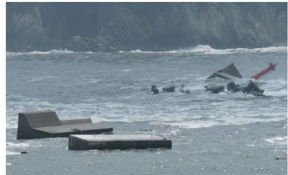
Fig. 6. Concrete debris from breakwater and seawalls offshore of Tarō, captured during the 2011 EEFIT mission.
