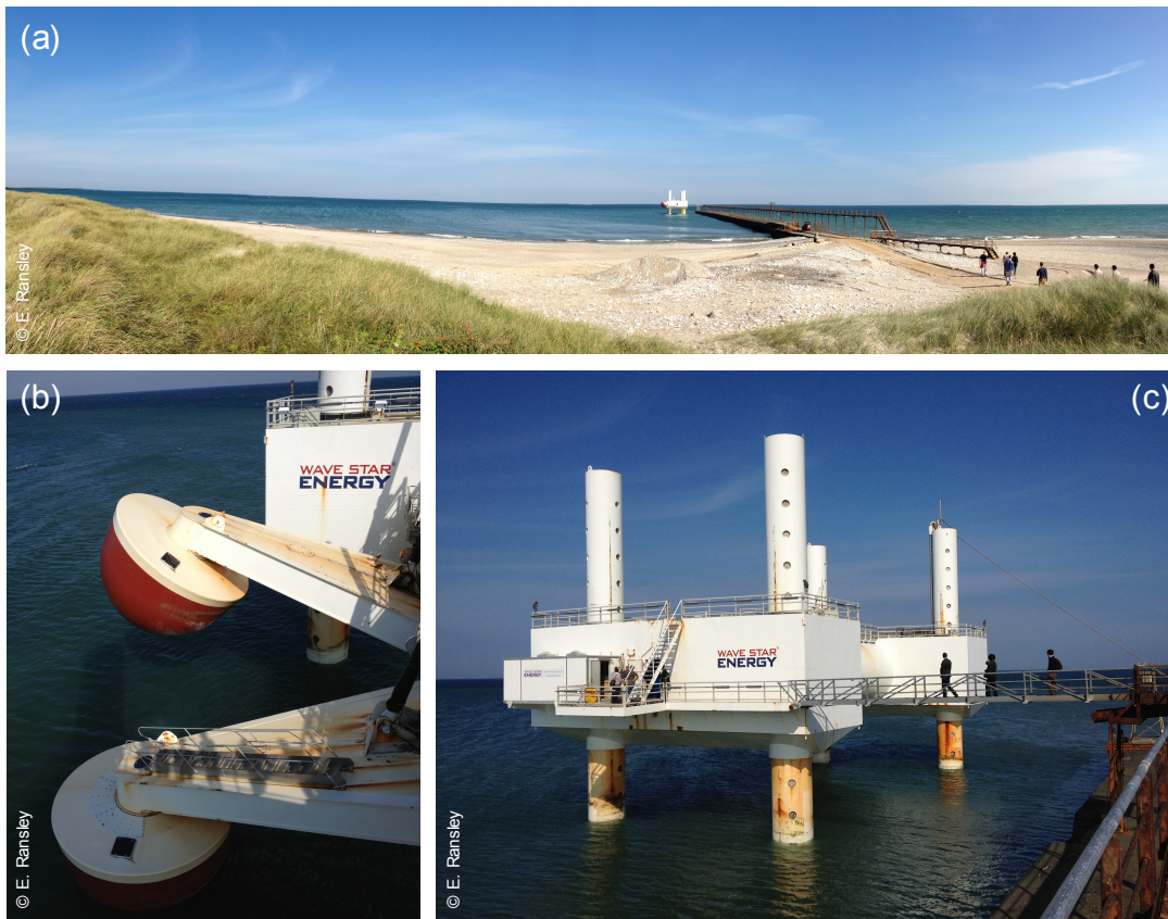
Figure 5.18: Photographs of the Wavestar prototype near Hanstholm, on the west coast of Denmark. Showing 2 point-absorbing floaters (b), the supporting platform and 4 monopile foundations (c). Photo Credit: E. Ransley (Sept. 2013).
