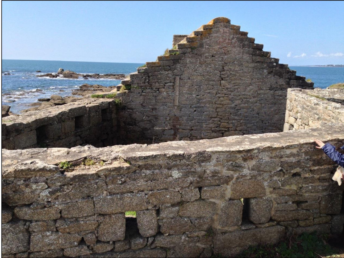
Plate 40 The ruins of the granite fort at Cabellou Point. Photo: C. Mansfield April 2014.
