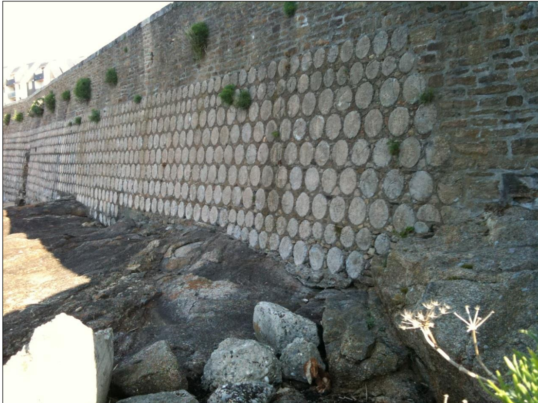
Plate 20 Spoiled cement barrels built into the sea-wall on the Russian Quay in Concarneau - photo Author's own fieldwork, C. Mansfield June 2010
