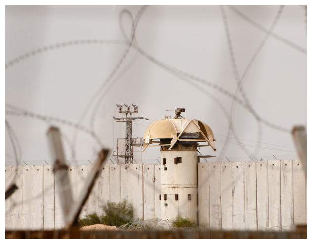
Remote-control gun tower, 'automatic kill zone' of the Israeli separation barrier, 2015. © Ryan Beiler.
