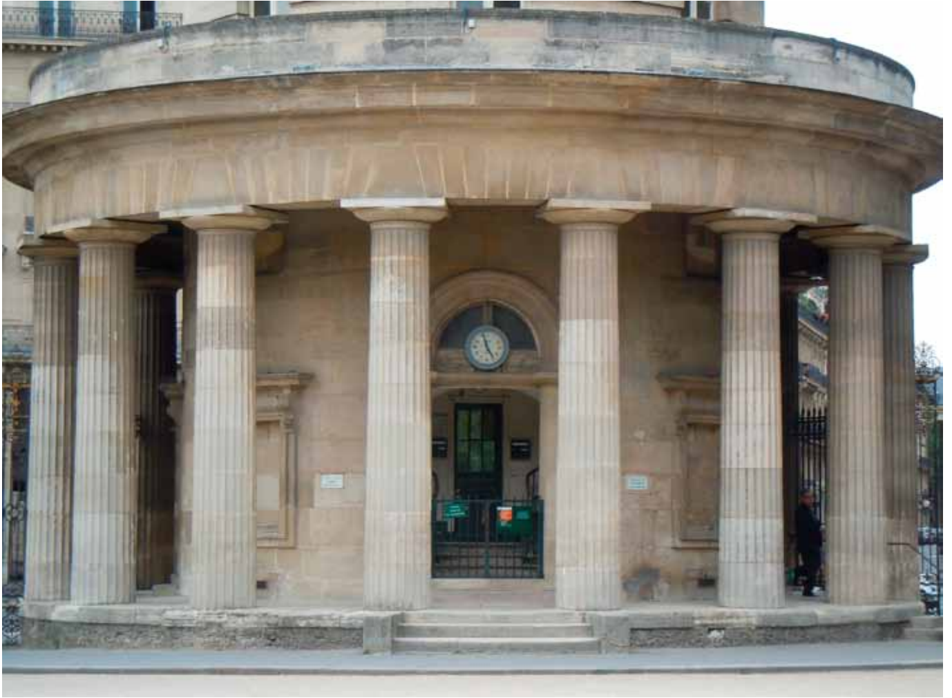
Figure 17.1 Claude Nicolas Ledoux, Rotonde (1787), part of the Farmers-General wall, Parc Monceau. Photograph: Uwe Bennert.
