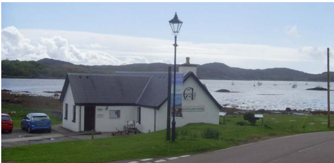
Figure 1. View of LSIC building, north facing entrance and reception and north gable wall of exhibition area.
