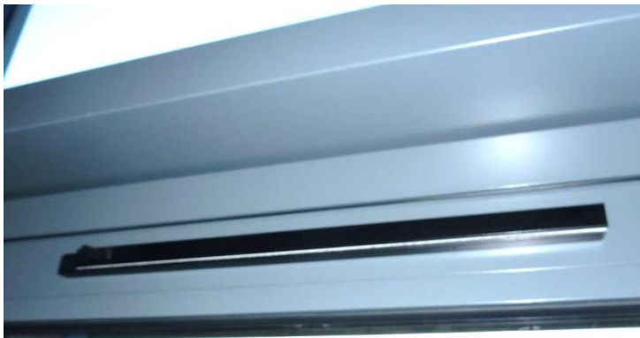
Figure 6. Trickle vent closed (Source: MEARU)
