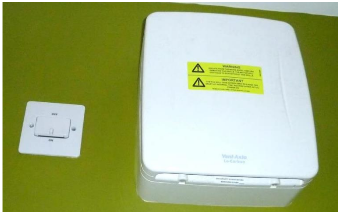
Figure 3. Mechanical extract fan turned off by building occupant (Source: MEARU)
