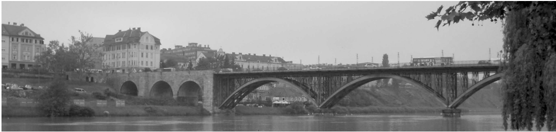
Fig. 2: The Old Drava Bridge, Maribor
