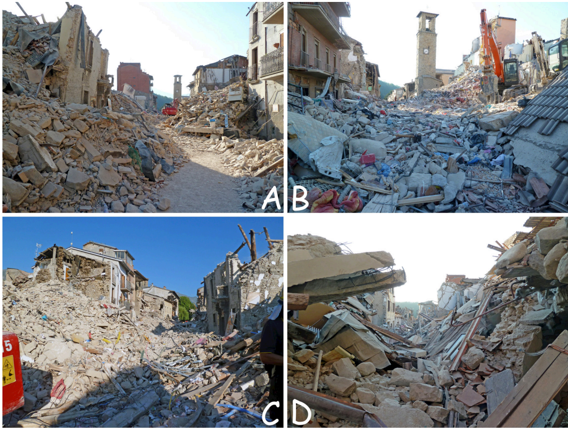
Figure 3. Views of the destroyed Amatrice downtown (10-11 MCS). A-C, Collapses of all the stone masonry buildings along Corso Umberto. Note that the only still-standing buildings are the Medieval tower (A-B) - which survived also to the 1639 earthquake - and a 5-storeys RC apartment building (A; this collapsed during the 30 October, M_w 6.5 earthquake). D, View of a road paralleling Corso Umberto, with almost complete destruction/collapse levels.
