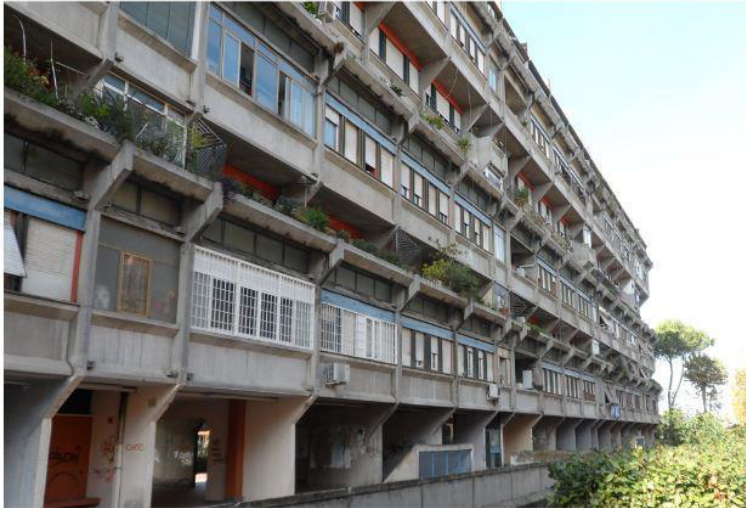
Fig.6. Facades in their current conditions.
