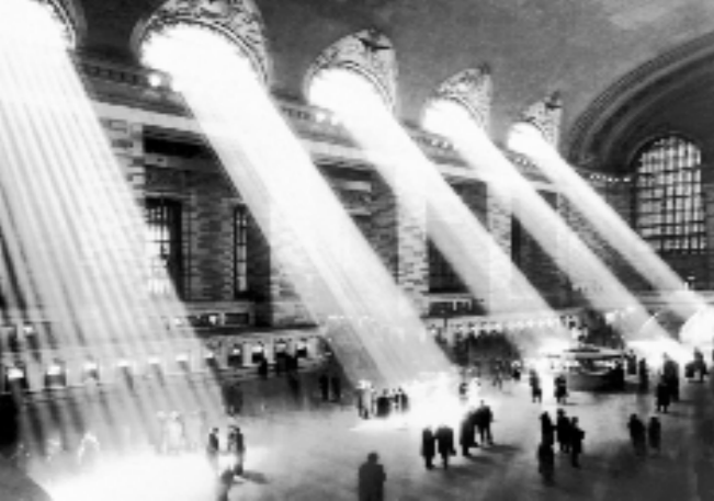
CENTRAL STATION NEW YORK_ 1962
