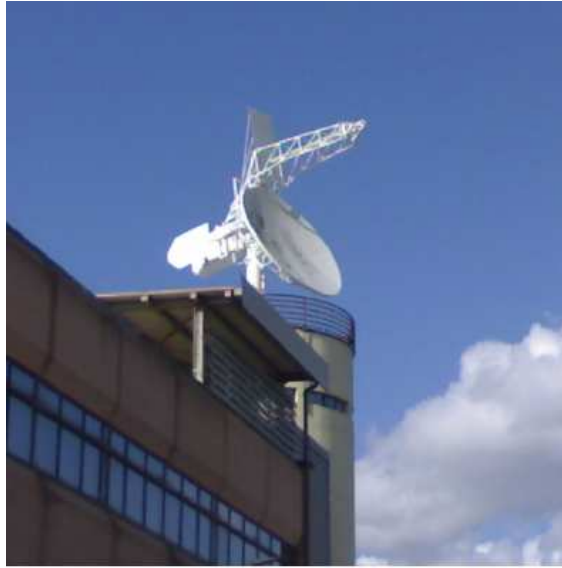
Figure 5.1 – Polar 55C antenna installed over the top of the building of ISAC, in the Tor Vergata Area of the National Council of the Research.
