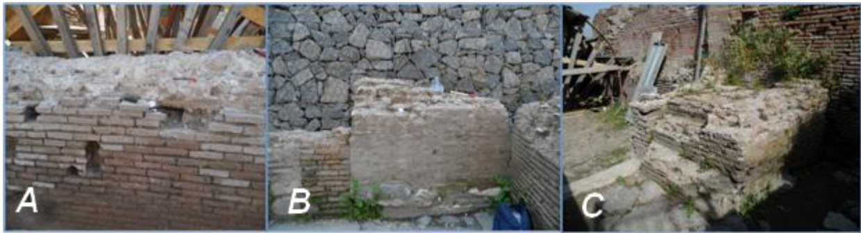
Figure 41. A visual check shows difference between structures where mortars were sampled. The picture B shows the wall owns to CMAX 6 and 7 and different from others in A and C pictures. Structures in A and C show the similar constructive technique called a lateritium.
