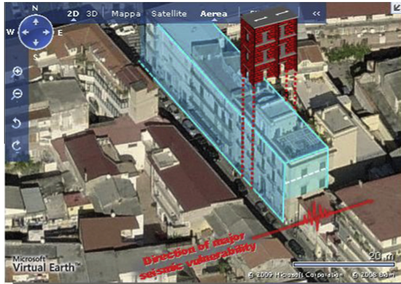
Fig. 13. Typical example of a structural unit extracted from a masonry building aggregate.
