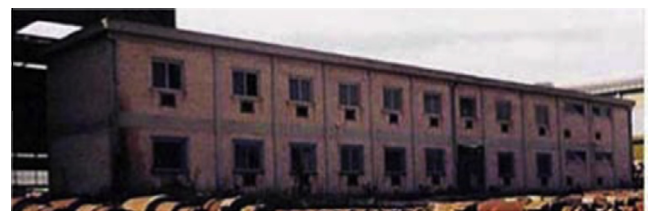
Fig. 1. The building tested within the ILVA-IDEM research project before experimentation.
