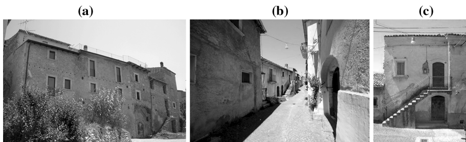
Fig. 1 South facade (a) and north facade, (b, c) of the modelled building aggregate located in San Pio delle Camere , Italy (Scheda di Aggregato 2010)
