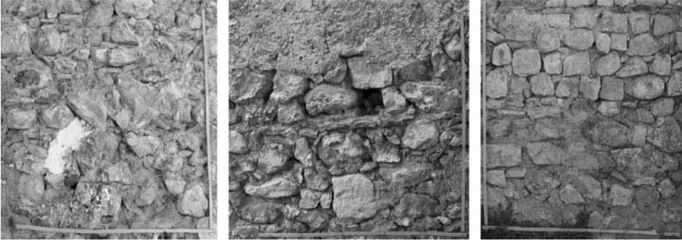
FIGURE 7 Typical masonry textures.
