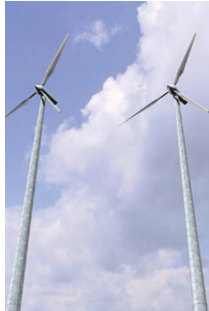
Figure 1: Examples of application of beams with thin-walled polygonal cross-section: (a) lighting tower; (b) mast for small-scale wind turbines.
