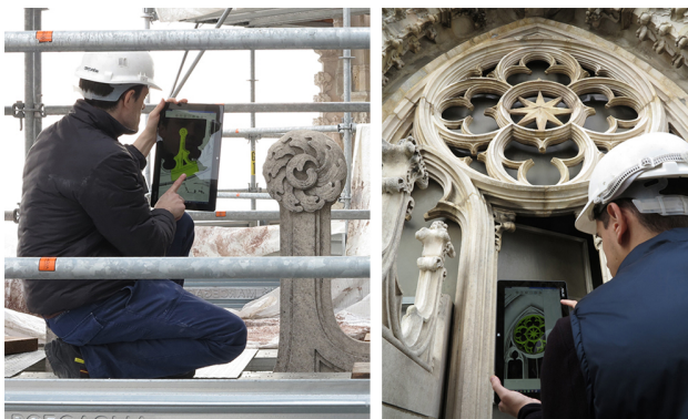
Figure 8. Use of BIM3DSG in the yard.
