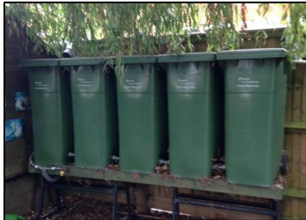
Figure 7.5: grey water and water butt system adopted
