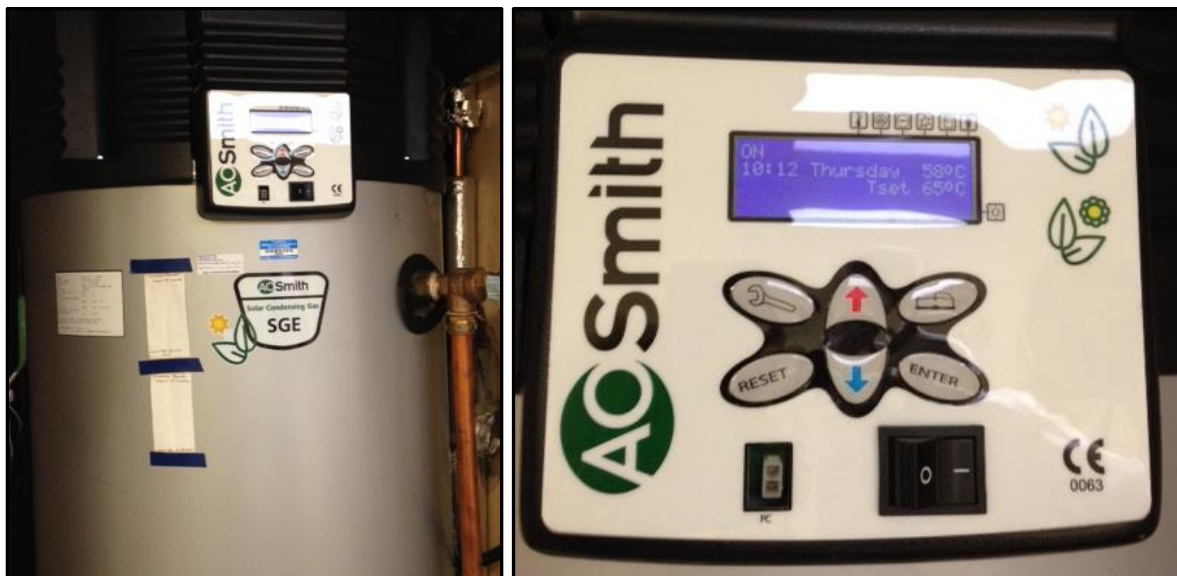
Figure 6.2: EEM (solar thermal system) adopted
