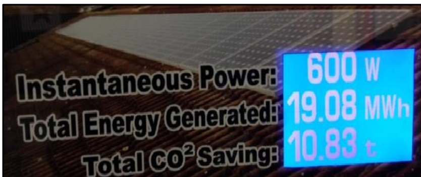
Figure 5.3: solar PV display unit
