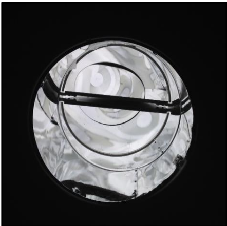
Figure 7.4: EEM (sun pipes) adopted
