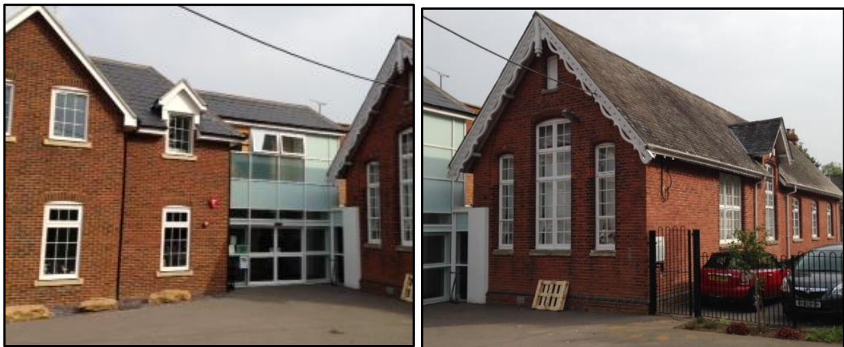
Figure 6.1: school retrofit project 3 site photos
