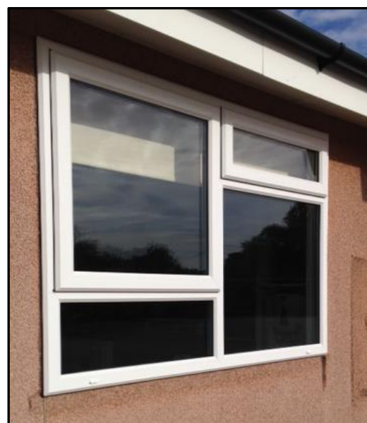
Figure 4.4: double glazing for project 1
