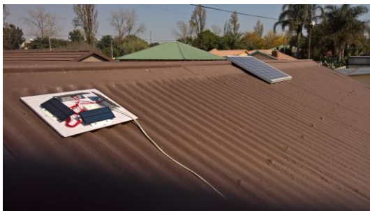
Figure 4: Left solar sensor, Right 50 W Solar panel
