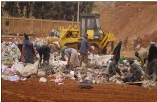
Fig. 3: Waste picking in Westonaria LM landfill site
