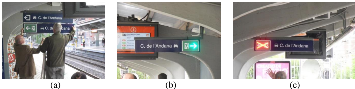
Figure 4: (a) The standard static exit sign, (b) the ADSS with flashing and running green arrow and (c) the ADSS with negating flashing red cross.
