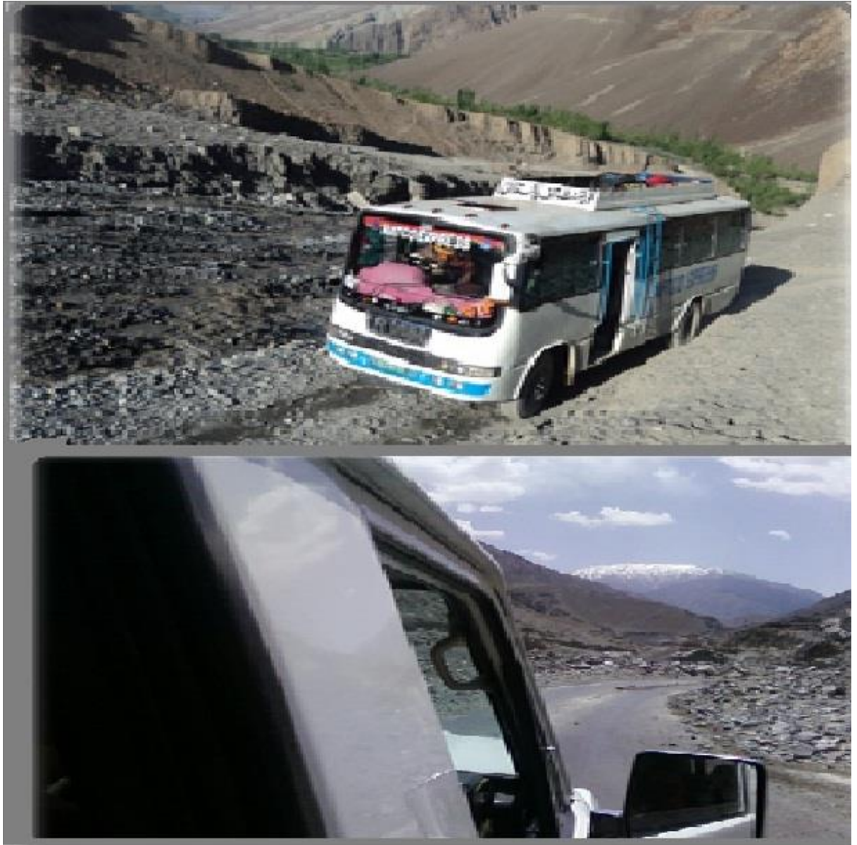
Figure 6.10 KKH [the Silk Route] Diامر: Land sliding (picture taken in May and June 2011) In (NATCO: Northern Areas Travel Corporation) is off the road due to the land slide.
