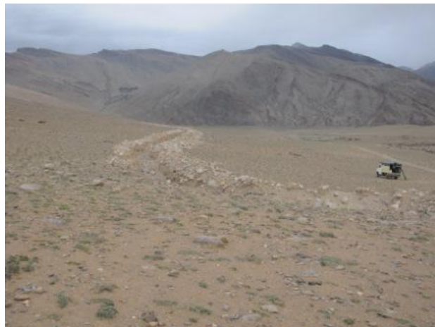
Fig. 9B: Excavated channel intended to carry water from the Zara river to Debring in the next valley to the east (photo: T. Stott).
