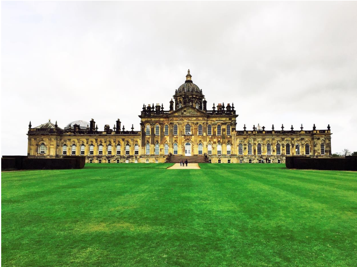
Fig. 4: Castle Howard, after restoration, South Face. Image reproduced by permission of Toby Lamarque.
