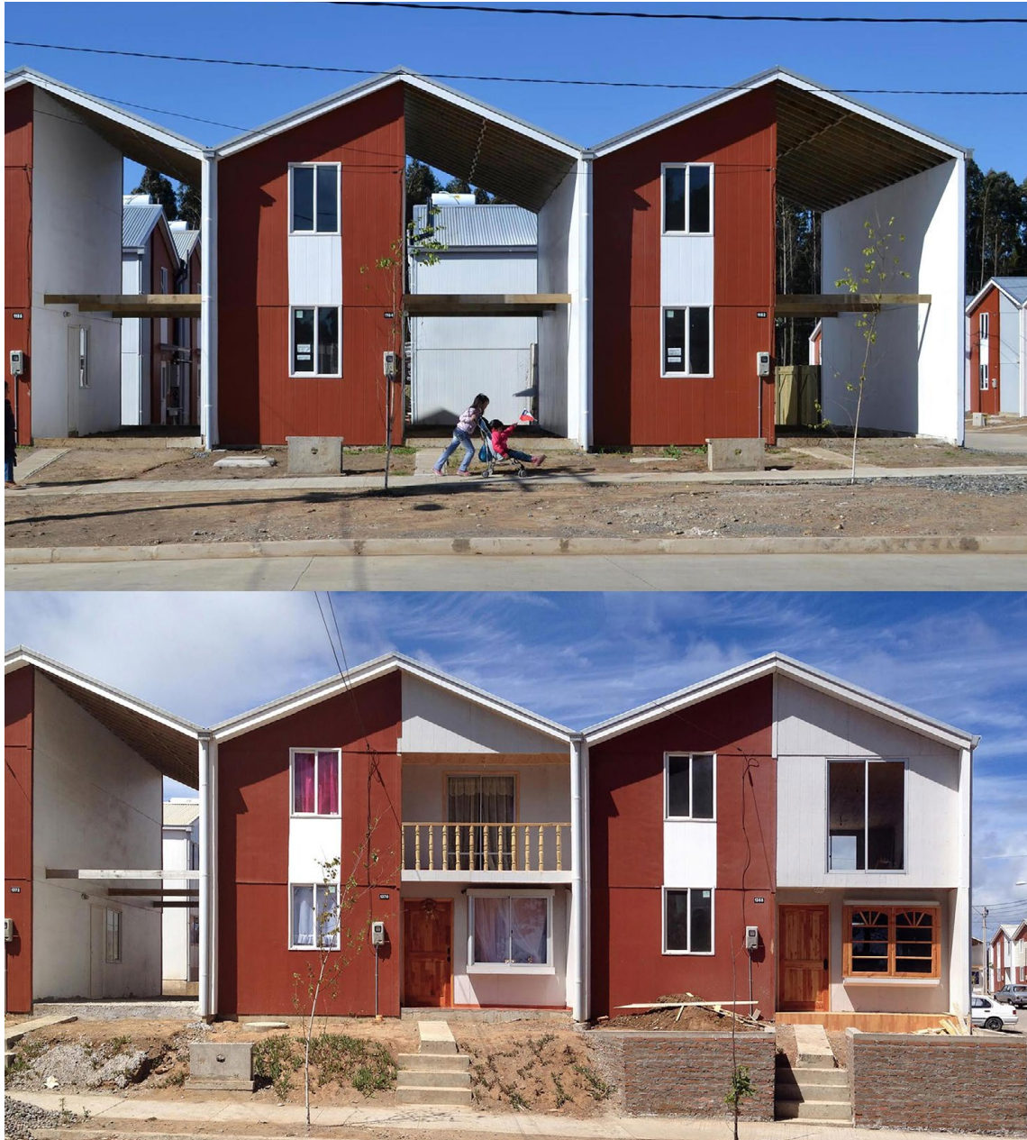
FIGURE 5. Villa Verde Housing - after 2010 Chile earthquake.
