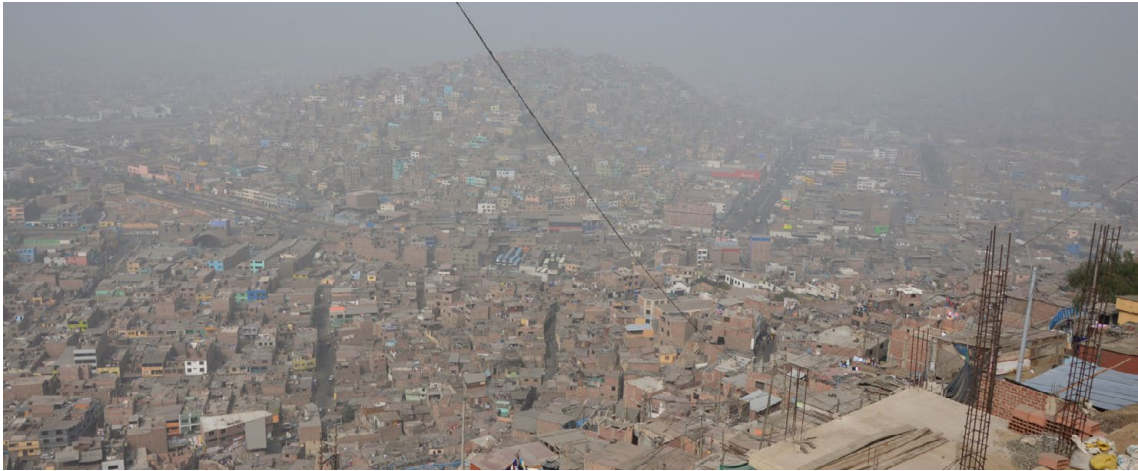
PICTURE 6. In the hill El Agustino new building structures are continually emerging both, as a part of a new home for a family to settle or as an implementation of a previous construction. Lima, Peru. Author: Maddalena Iovene
