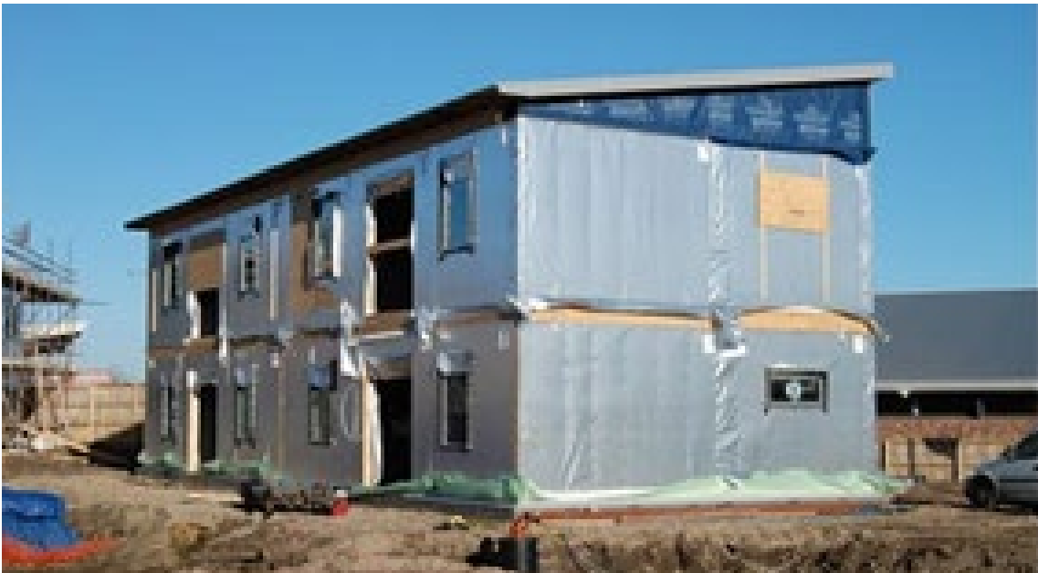
Image 03. BoKlok Generation 1 Apartments timber framing system under construction (Image: D.Morton)
