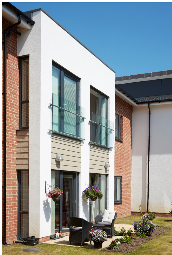
Figure 1: State-of-the-art accommodation for older people
