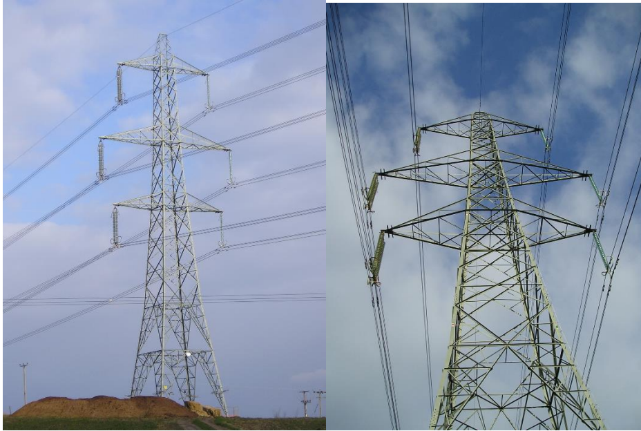
Figure 3: D L6 Blaw Knox type suspension tower located in Dorset, UK (Hendry, 2005)
