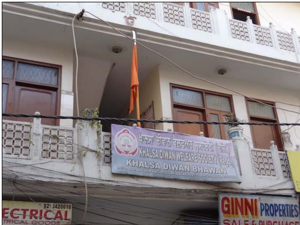
Figure 1: Offices of the Khalsa Diwan in West Delhi
