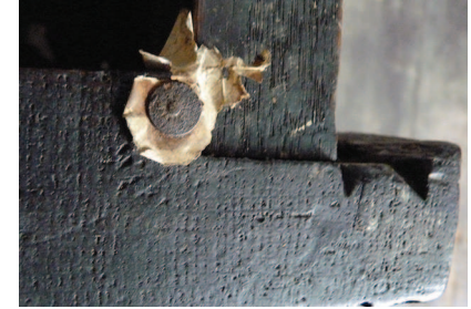
Fig. 10 Stile showing horn-like indentations, Canterbury.
