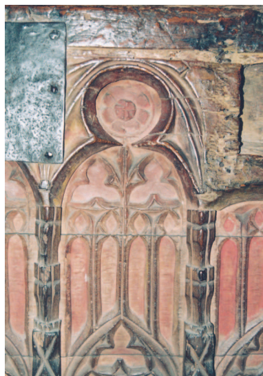
Fig. 21. Detail of arcading showing colour, Faversham.
