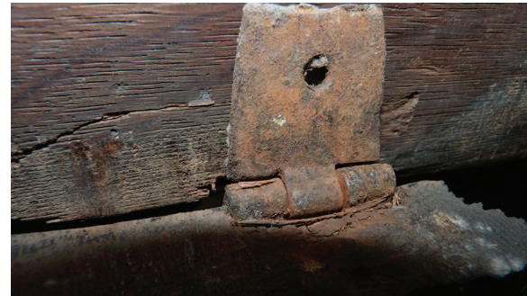
Fig. 17 Example of mortised knuckle hinge with flange out of mortise, Norwich.
