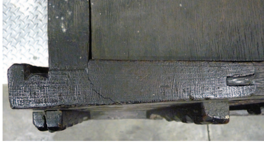
Fig 8 Stile showing tapered section, Norwich.
