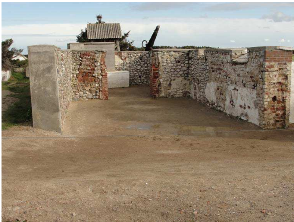
Figure 4. Mårup Church after its “creative dismantling” in 2007.
