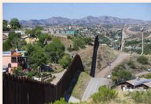
Figure 9: Example of steel fence enforcing border division [28].
