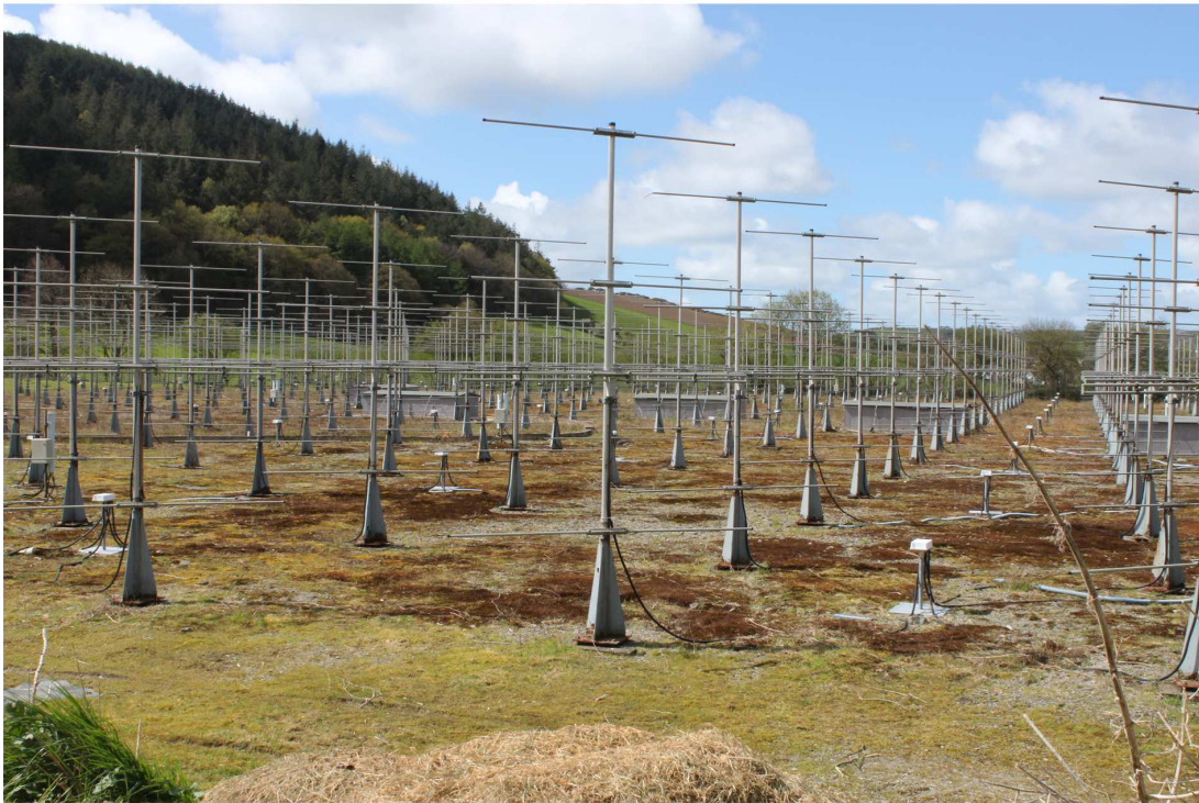
Figure 2.9 The 46.6 MHz NERC Mesospheric Stratospheric and Tropospheric Radar at Aberystwyth, West Wales, United Kingdom.
