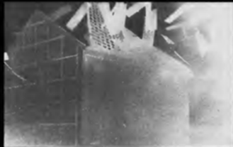
47 kt Greenhouse Easy, Eniwetok Atoll, 1951. Brick house, 3 psi peak overpressure
