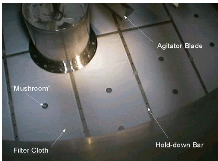
Figure 6.3: Internal view of filter 24/970
