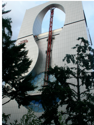
Insert figure 9.1 (the namBa HIPS building, Osaka, photograph by the author)
