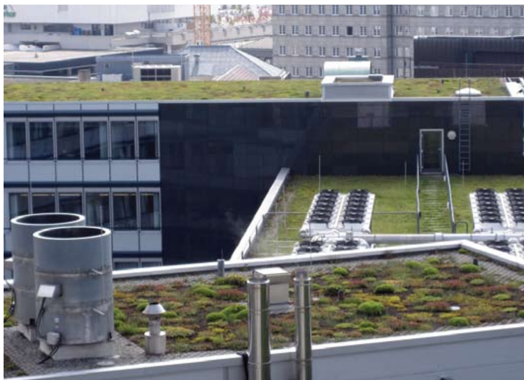
Figure 10: Green roofs are a key component for mitigation of the urban heat island effect in city centres. Source: Authors
