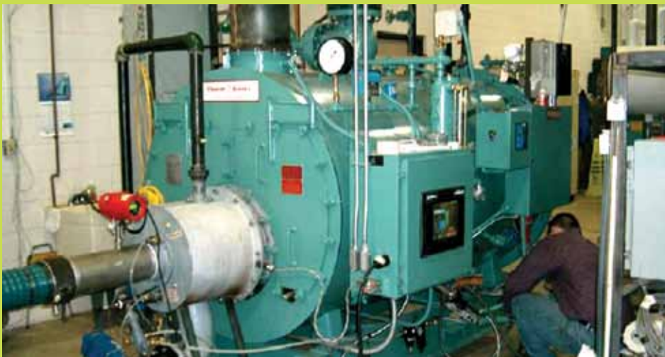
ပုံ ၃ Two-stage Super Boiler [5]
