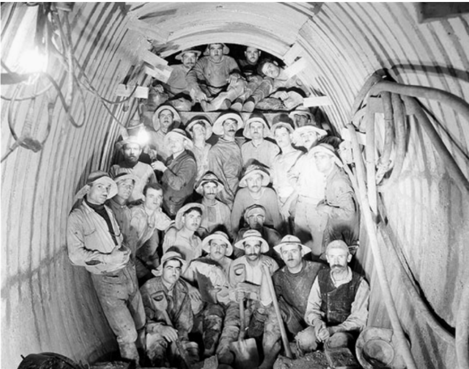
Figure 7. Male labor was reserved for the “harder” tasks involved in the construction works. (Source: Photographic archive, Water Supply and Sewerage Corporation of Athens 1995)
