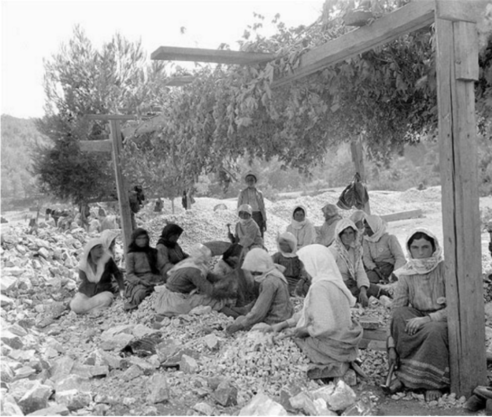
Figure 6. Female labor was used for the “easy” task of veneering the dam with marble. (Source: Photographic archive, Water Supply and Sewerage Corporation of Athens 1995)
