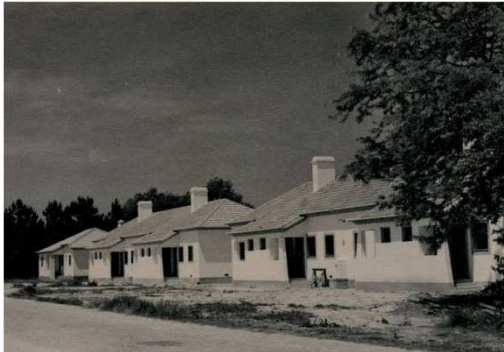
Figure 8: House of Guarda de Pedreanes
