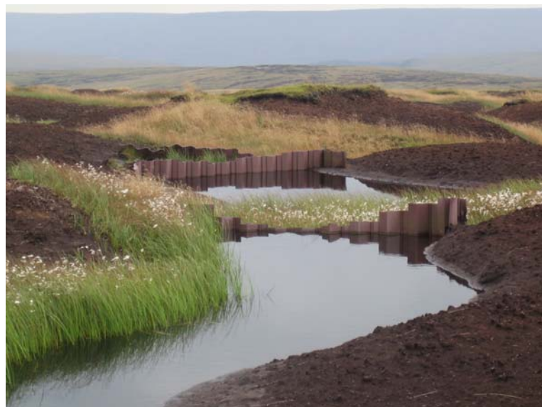
Figure 5.2: Gully-blocking on Bleaklow to raise the water table, trap peat sediment and encourage colonisation by cotton grass and other blanket bog species. Such activities should reduce fire risk (Photograph ©Julia McMorrow).
